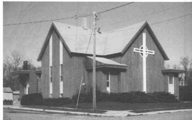
Methodist Church—Elma—after 1961 remodeling.
